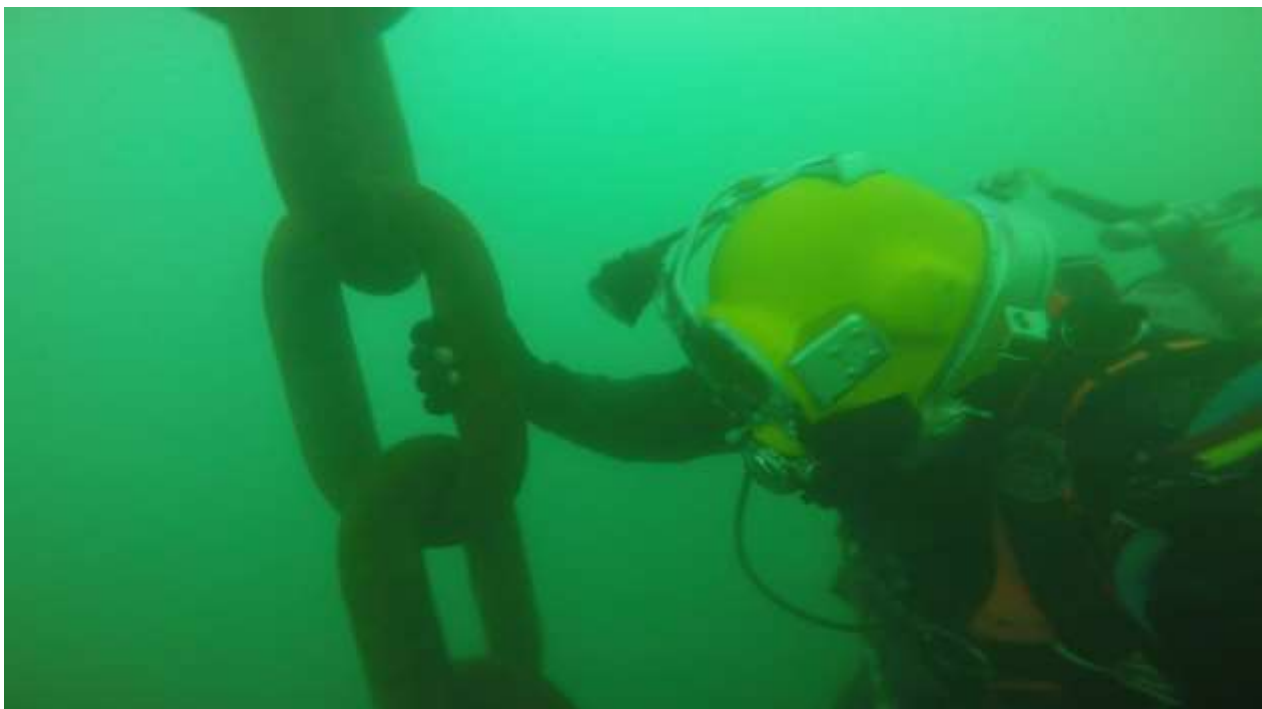
Divers Inspect Main Stream Mooring Chains
