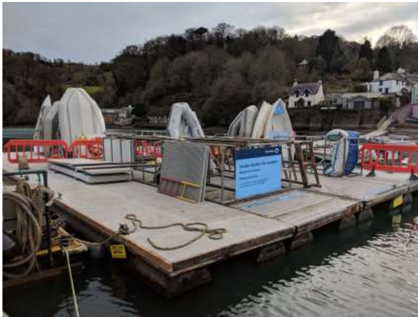
Fig 3 – Dittisham Pontoon Decking Replacement
