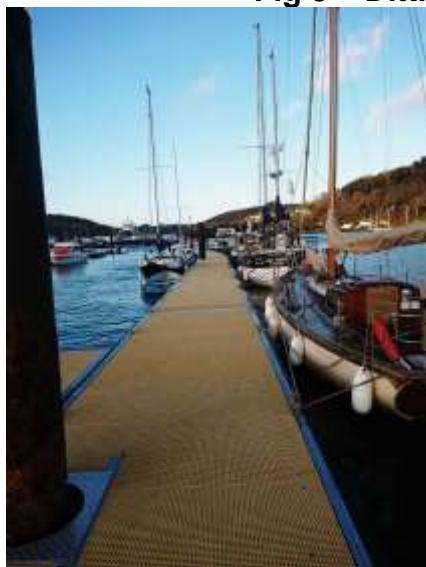
Fig 3 – Replacement DA Pontoon
