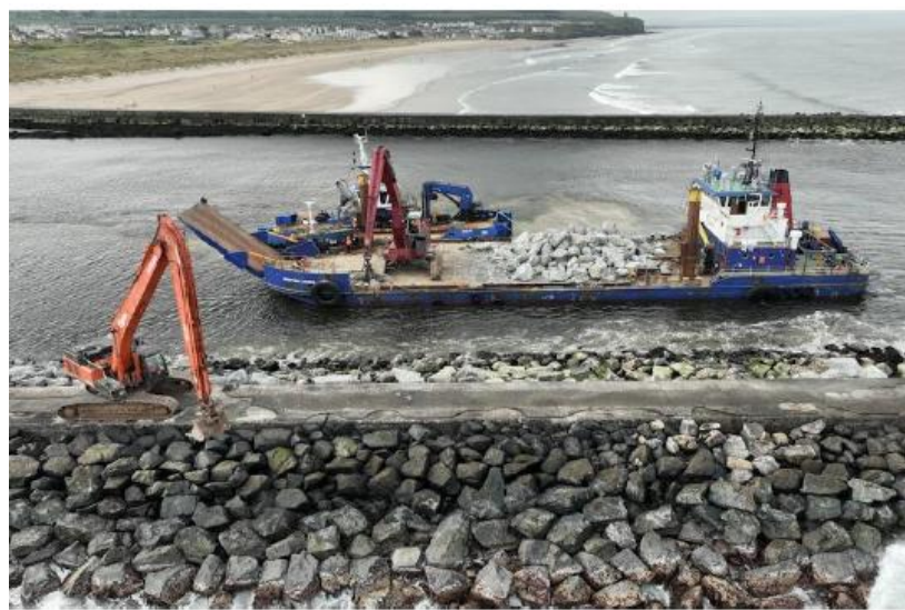
Stephen James off-loading 1-3T rock armour on a project.
